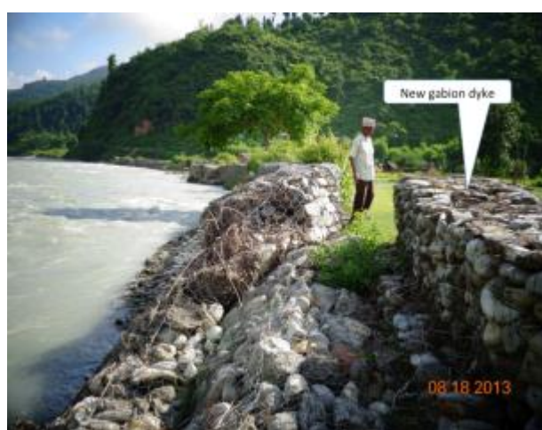
Figure 14 Bank protection works along Budhiganga river at Sisnephat
