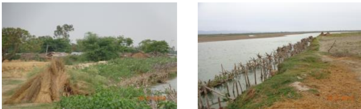
Figure 7 Bamboo porcupines and bioengineering works along right bank of West Rapti river near Holiya
