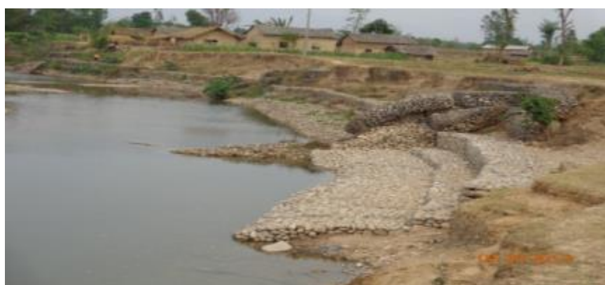
Figure 11 Bank protection works Man Khola river at Naudasta
