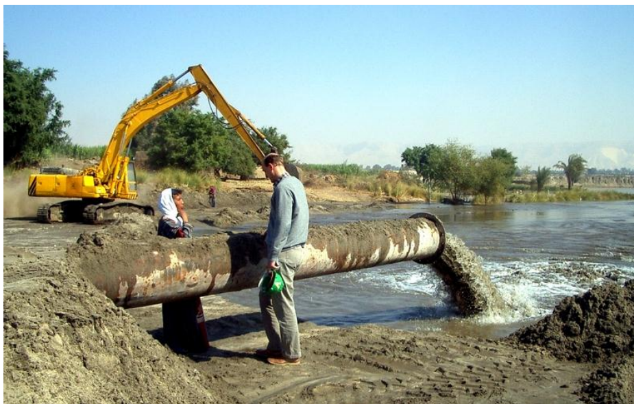
Figure 2.5: Pumping sediments from River Nile for land reclamation for agriculture, Egypt 2006
