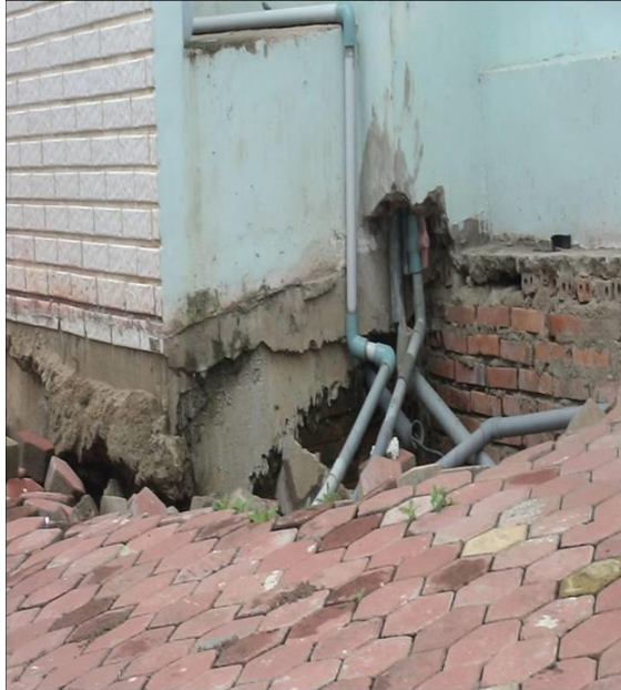
House Foundation Failure due to Land Subsidence
