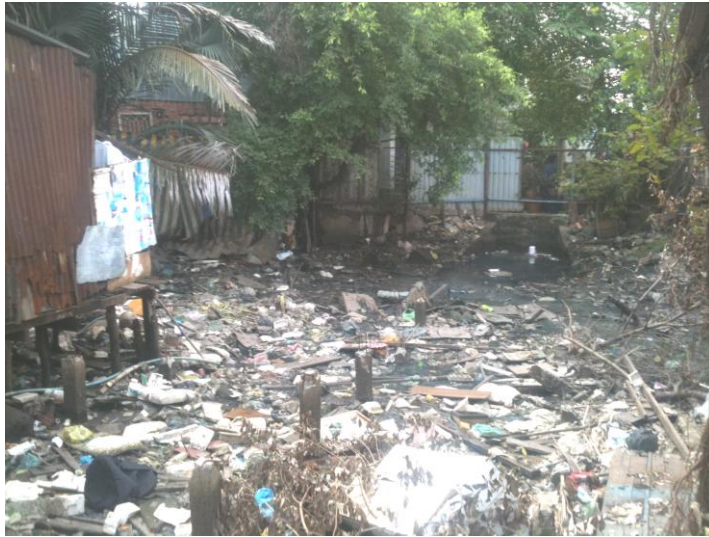
Wastes Block Natural Drain Channel in Ho Chi Minh City
