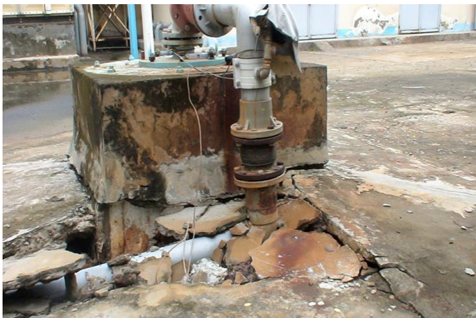
Land Subsidence around a Tube Well in Ho Chi Minh City
