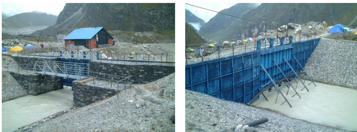
Figure 8. Open canal of Tsho Rolpa Glacial Lake, and iron gate on the open canal
