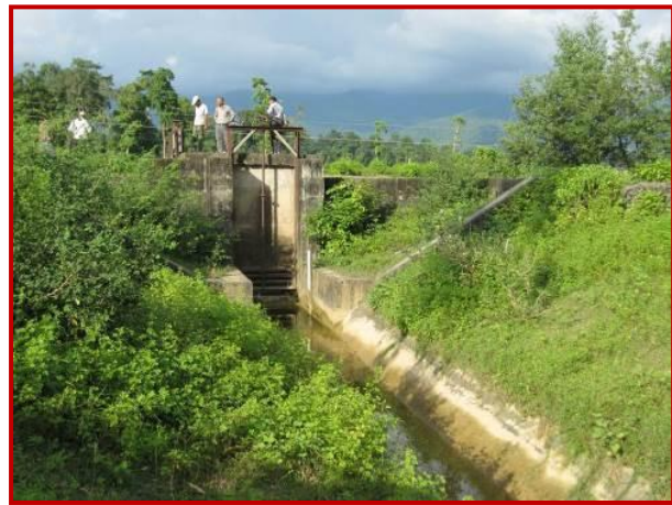
Photo 3-2 Failure of Diversion Core Wall Photo 3.3: Headworks Gate into Lined Main Canal Constructed across the River
