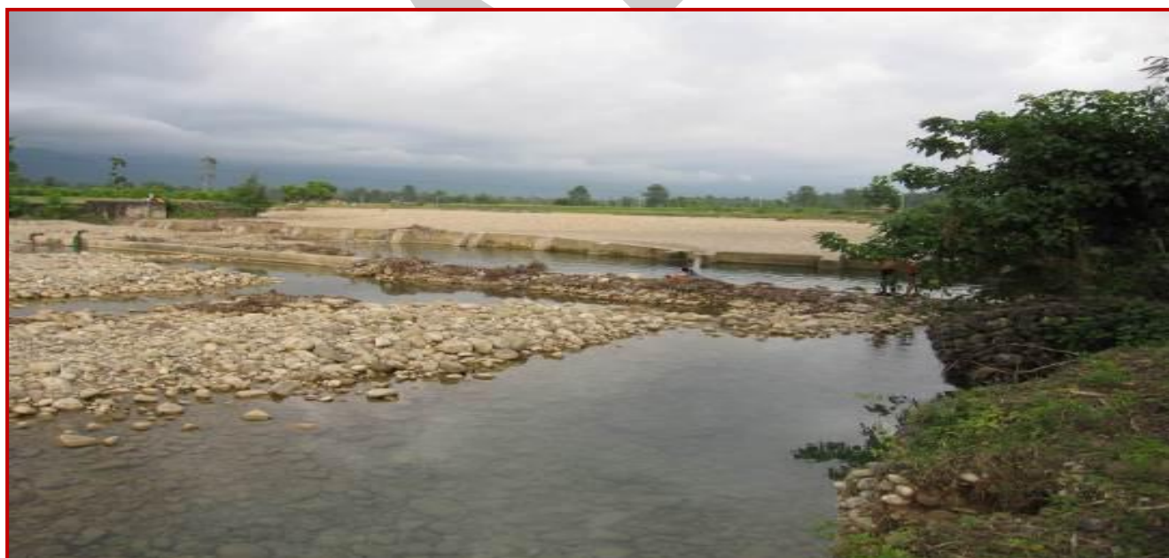
Photo: 3.1 Core and Cut-off Walls across Man Khola
