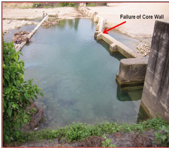
Photo 3-2 Failure of Diversion Core Wall Photo 3.3: Headworks Gate into Lined Main Canal Constructed across the River
