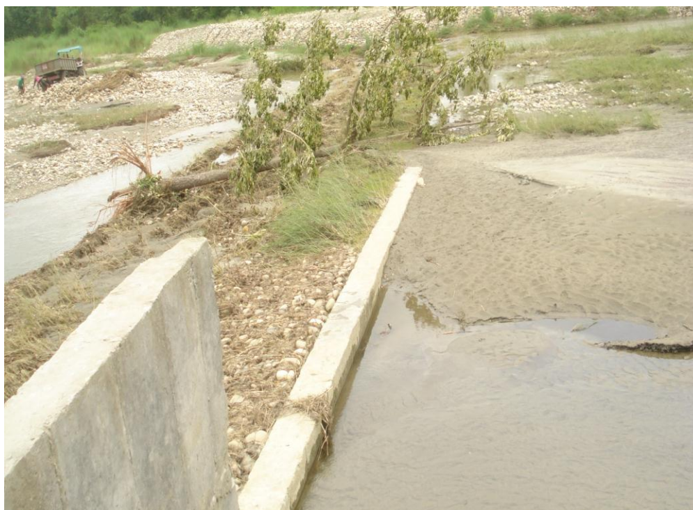
Photo 3.6: Orifice Type Canal Intake with Trash rack
