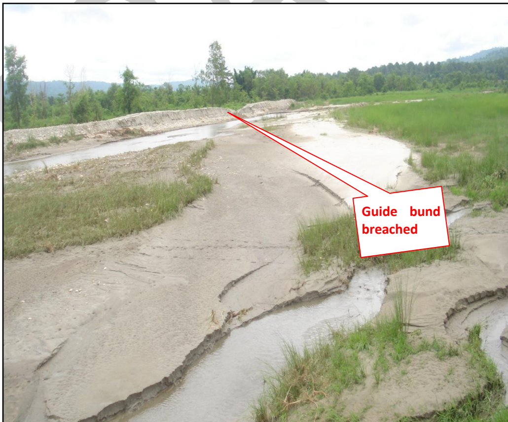
Photo 3.8: Guide Bund Breached and shows catchment area at U/S side
