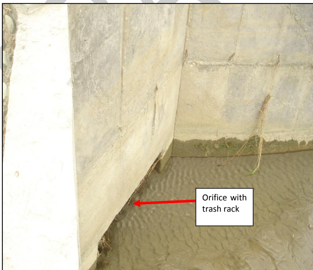
Photo 3.6: Orifice Type Canal Intake with Trash rack
