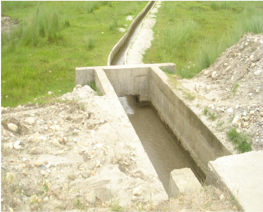
Photo 3.7: Intake Structure with Sediment Trap
