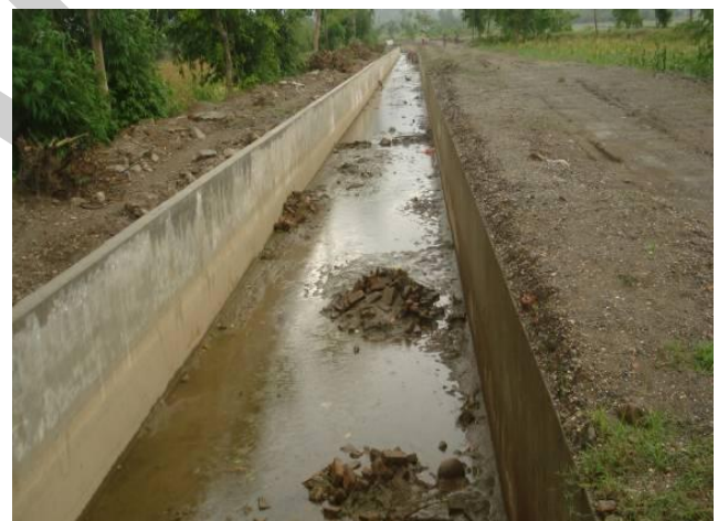
Photo: 3.4 Brick Lined Canal Over Designed Section
