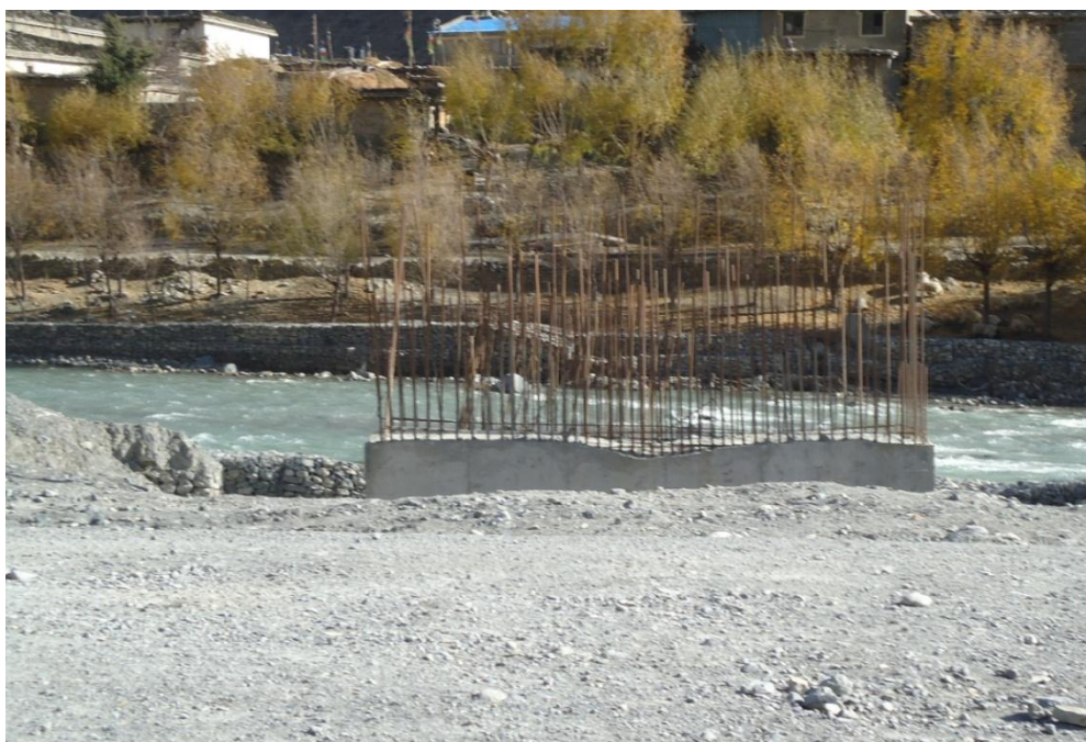
Fig. 5a: Bridge axis. The photo was taken from location of right abutment. The contractor has completed the foundation of the pier. Other works are still not started.
