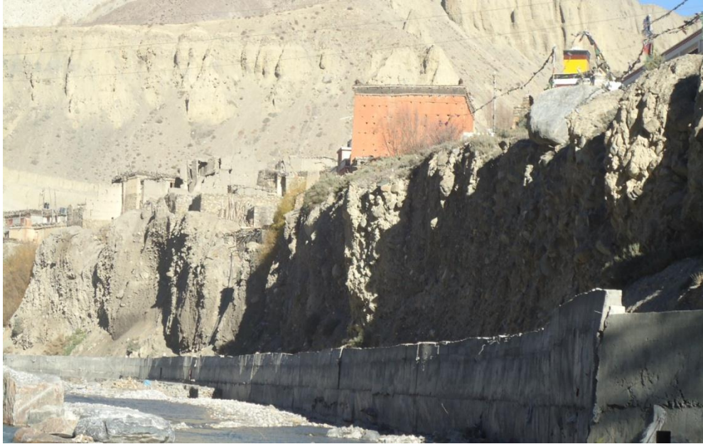
Fig. 6a: Photo showing bank protection wall at upstream from the confluence of Kaligandaki River and Kag Khola. It is a concrete wall and is located at left bank of Kaligandaki River. Concrete walls are rarely used for bank protection works in Nepal. Generally they are made of gabions. It is to be noted that such concrete wall can be replicated at other locations if its performance will be satisfactory.
