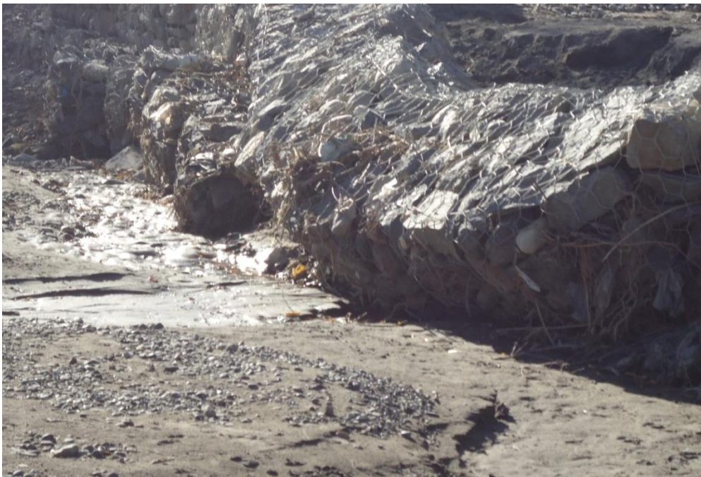
Fig. 5c: Collapse of gabion protection works at right bank. Protection walls at both banks are damaged at several locations. These walls were constructed by DDC/local people.
