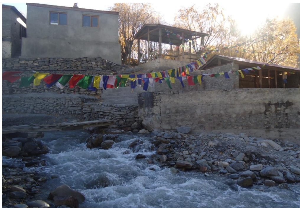
Fig. 6 c: Gabion protection walls are provided along both banks of Kag Khola to protect the Kagbeni settlement. The walls are damaged at several locations due to steep river slope.
