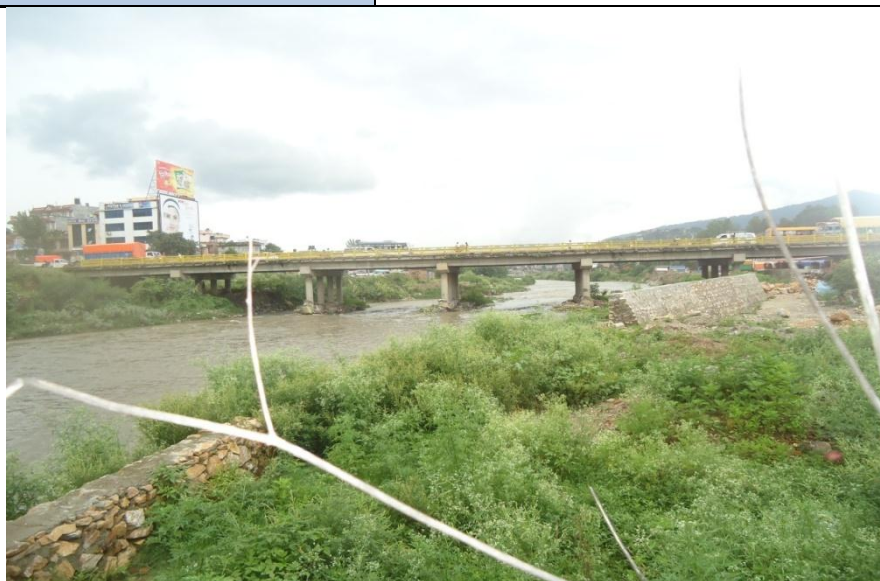
5a: General view of the bridge from upstream. It is a RCC T beam bridge on pile foundation. The bridge has 5 spans and its total length is 90m
