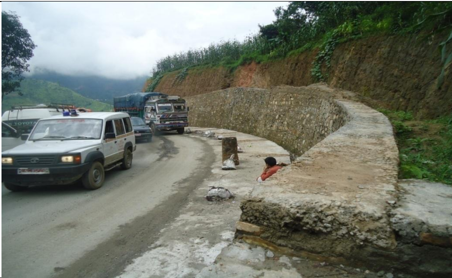
Fig. 4b: Starting point of widening (towards Kathmandu side). Most of the road section is widened by excavating hill side and providing stone masonry breast wall.
