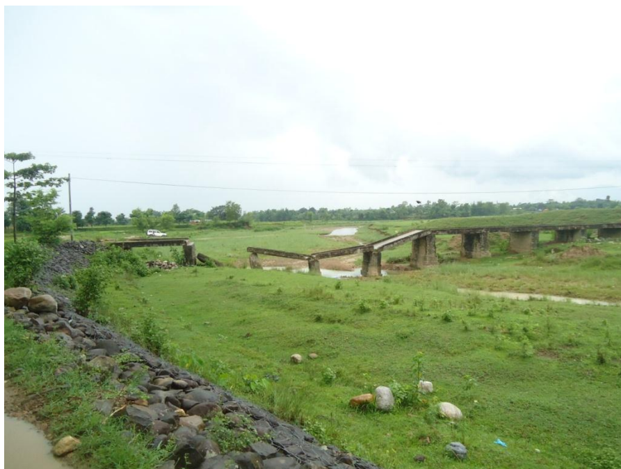
Fig. 4a: Photograph of the damaged bridge from the left bank. As seen, the bridge has collapsed due to settlement of piers.
