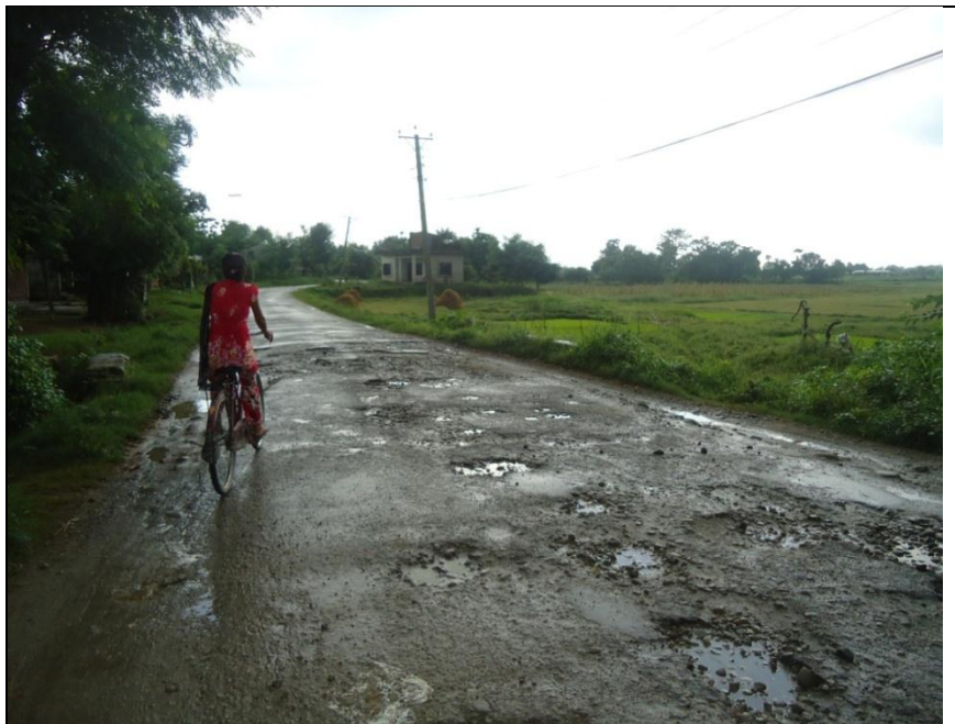
4b: Damage to the road pavement due to accumulation of water for a long period.
