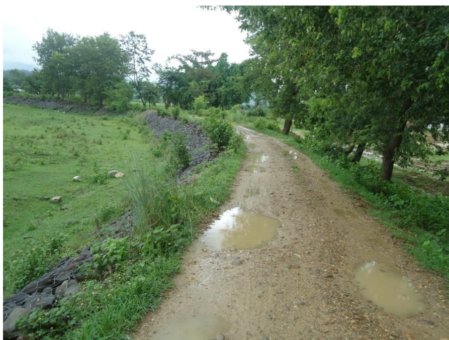
Fig. 4c: Earthen embankment is constructed at the left bank to regulate the river course through the bridge and protect the farm land. As seen on photo, the river is in bend. Due to the bend, the river is scouring at left bank and causing silting on right bank.
