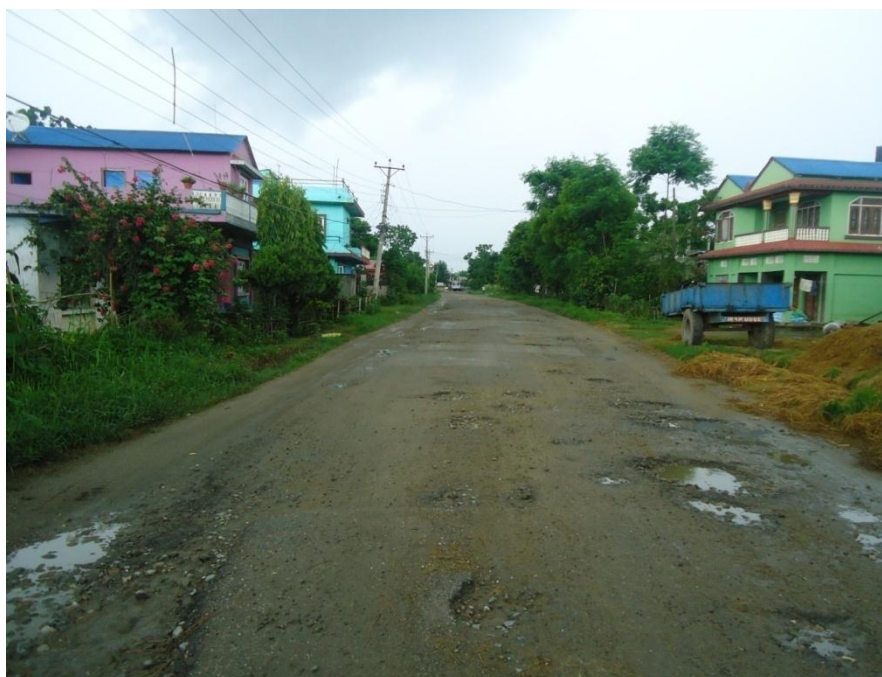
Fig. 4c: Houses are constructed at both sides of the road without provisioning of side drains.
