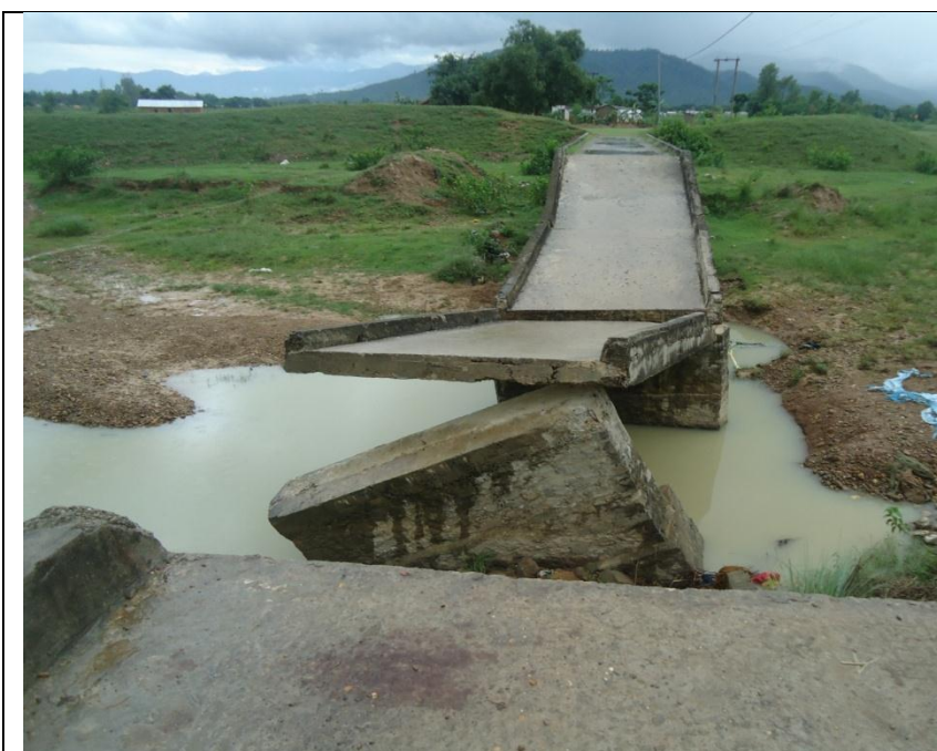
4 b: View of damaged portion of the culvert from the left abutment. As seen, the pier has completely settled and the concrete slabs are displaced/missing.
