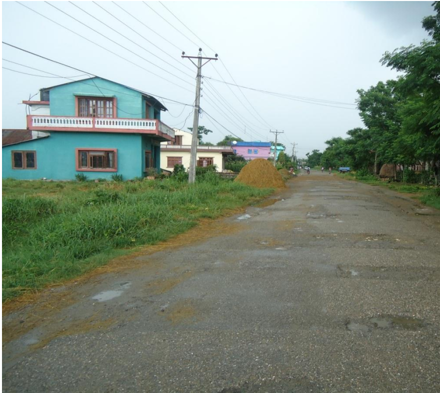
Fig. 4a: Starting point of Gitanagar settlement. There is no side drains at both sides.
