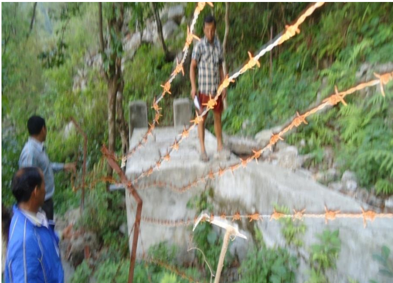
Fig. 4b: Small RCC intake of about 2m long, 1m wide and 1.5m high. This intake is meant for small water supply system which serves about 50-60 houses. During rainy season when the discharge in the source is high, excess water overflow from the tank and make the area very wet and unstable. This phenomenon is also one of the main causes of the landslide.
