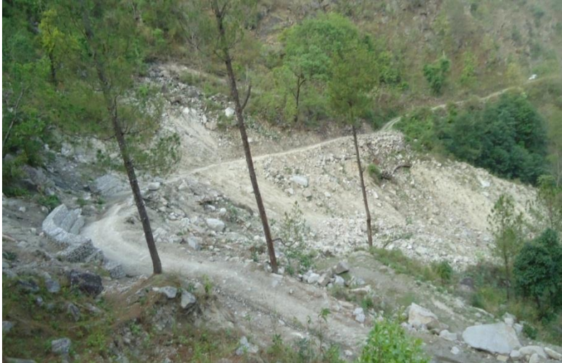
Fig. 4a: Photo covering the total area of the landslide and the damaged portion of the road. As seen on photo, the slope consists of loose loose gravels and materials mixed with boulders which is very susceptible to landslide. Gabion breast wall is provided at the middle of the landslide.
