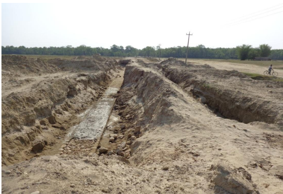
Fig. 4a: Rapti River has washed away a road section of left approach road. The washed away section is about 200m from the bridge towards Baghouda side. DoR has planned to construct a 20 m long Bailey Bridge at this location. The steel truss bridge across Rapti River can also be seen on photo.
