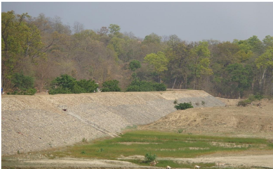
5c: View of the dyke from intake. The river side slope of the dyke is protected by gabion mattress and stone rip rap. It condition is good.
