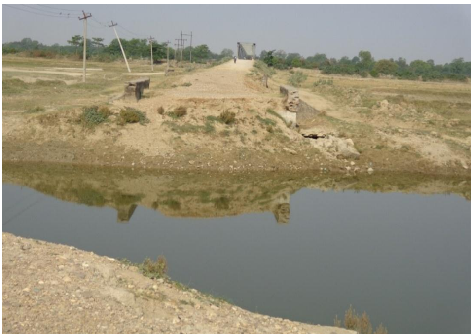
Fig. 4a: Rapti River has washed away a road section of left approach road. The washed away section is about 200m from the bridge towards Baghouda side. DoR has planned to construct a 20 m long Bailey Bridge at this location. The steel truss bridge across Rapti River can also be seen on photo.
