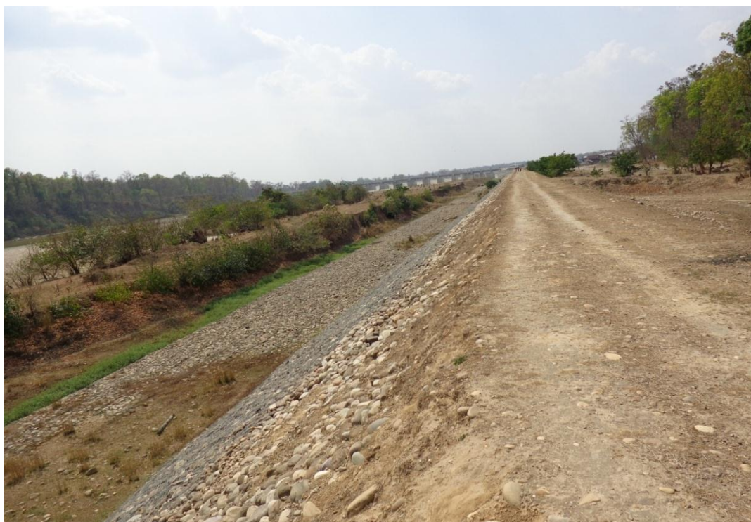
5a: Photo of dyke. It is an earthen dyke of about 4-5 m height. The top width of the dyke is 3 m. At the river side (left side) the slope is protected by gabion mattress at the lower portion and by stone rip rap at the top. Gabion mattress (launching apron) is provided at the bed for protection against scouring.
