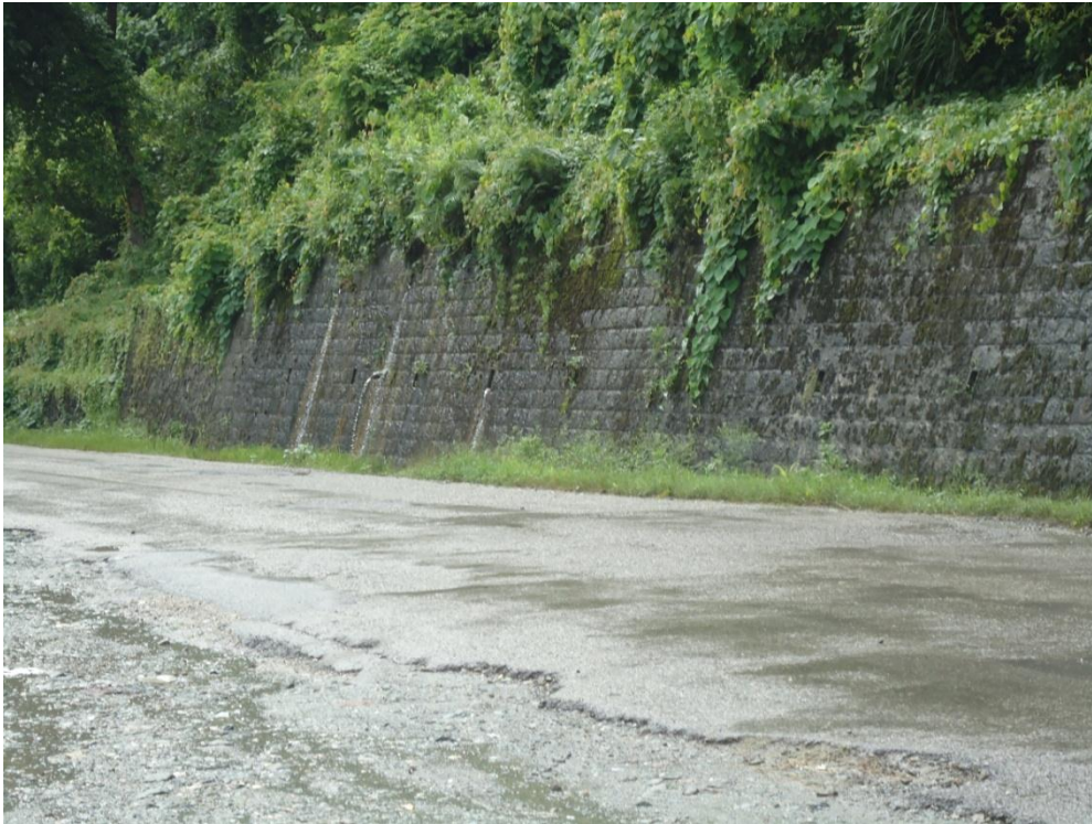
5d: Stone masonry breast wall near the bridge. As seen, substantial amount of water is coming out of the weep holes. Such water sprouts indicate that the slope is very wet. Landslides are very common on such wet slopes.
