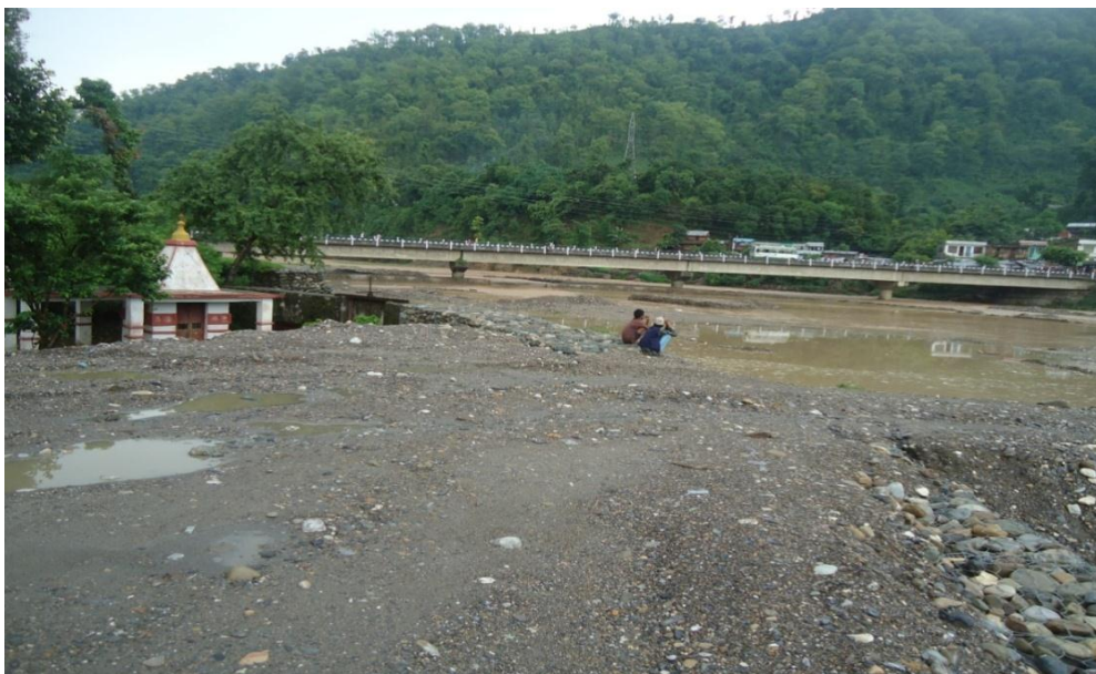
4b: View of the bridge from the dyke at right bank, downstream. The elevation of the adjoining village at this side is less than that of river bed level (see the level of the temple). DoR has constructed a long dyke to protect the village
