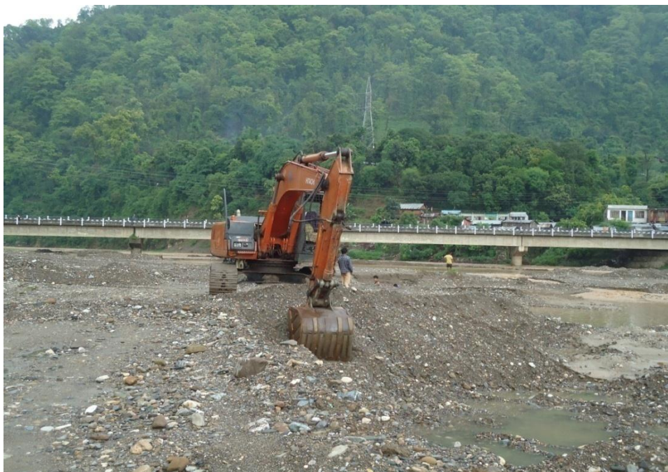
Fig. 4d: Photo showing excavaton of river bed materials at downstream. DDC contracted to a private company to extract the river bed from the bridge site to lower the river bed level. However, the speed of extraction is very slow.
