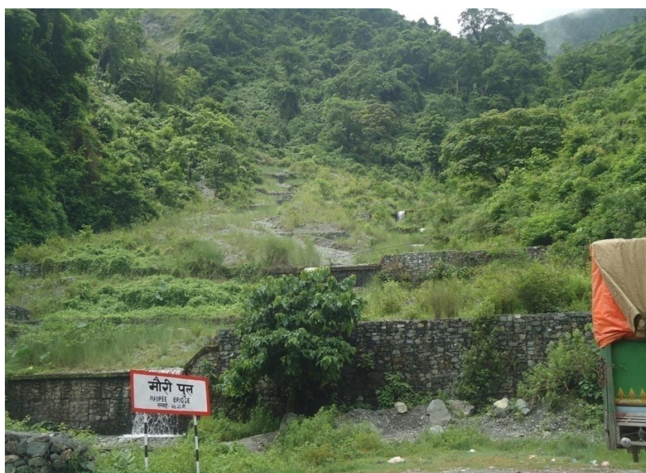
5a: Photo showing series of check dams at hill side of the road. As seen on photo, the check dam starts from the immediate hill slope of the road and extends to about 150m upstream.
