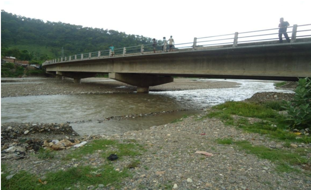
Fig. 4a: Extensive siltation near/at the bridge site. Difference between bed level and bridge is reduced to 2.5 m which was 8m in 1978. This shows bed level has risen by 6m within the span of 35 years. If the situation is not controlled the bridge will be washed away in future
