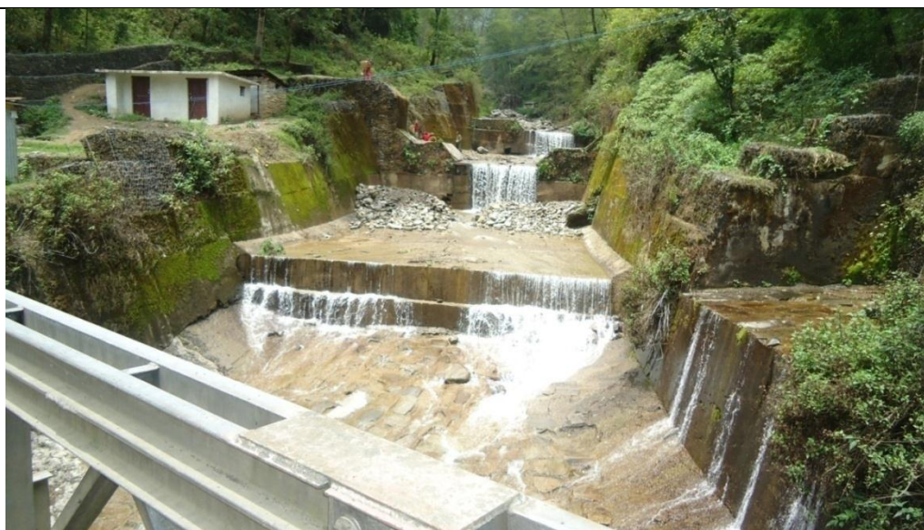
Fig. 4b: Upstream side of the river from the bridge. Several drop structures as along with concrete aprons are constructed at upstream as well as downstream to lessen the velocity of the river.
