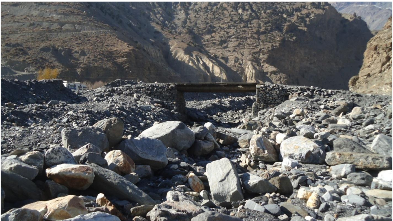
Fig. 4b: Timber bridge along the existing temporary crossing. Due to washing away of the road sections, temporary road crossing is built at about 200m downstream of the previous road alignment.
