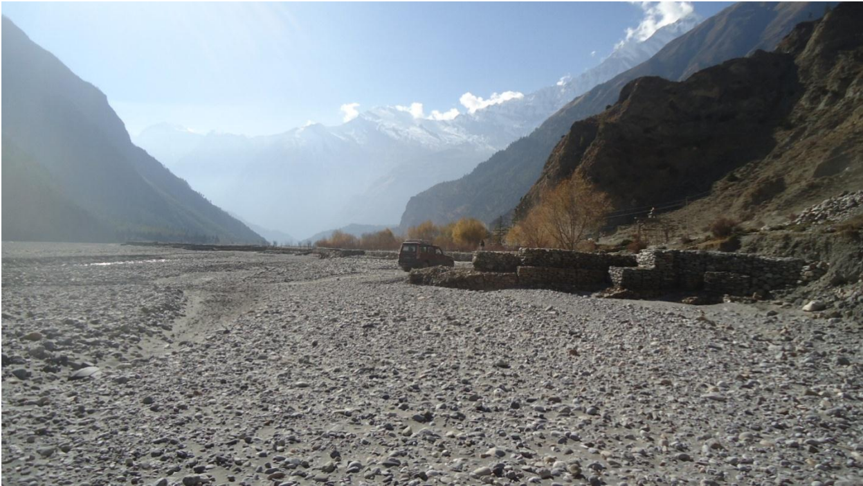
Fig. 5c: Series of spurs are provided at about 60 m downstream from the damaged road to protect the bank from river erosion. About 1.5 km long right bank at this area is highly vulnerable to erosion.
