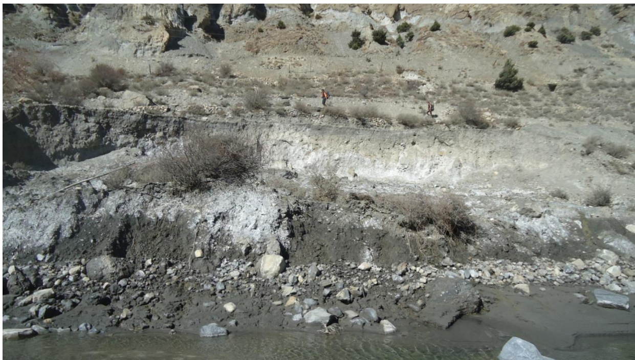
Fig. 5b: Photo of damaged road from the river side. The newly constructed road is about 10m away from it.
