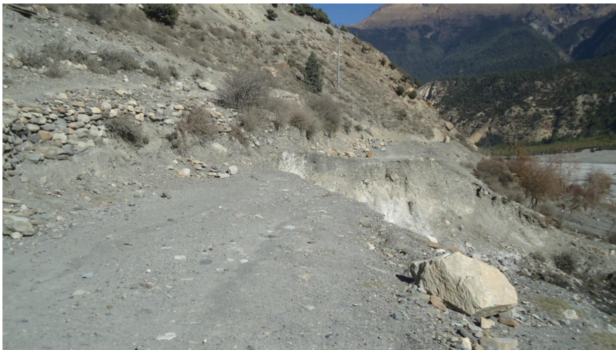
Fig. 5a: Washing away of road section due to heavy erosion. DoR has constructed a new motorable track at hill side. However the newly constructed road may be damaged if it is not protected.
