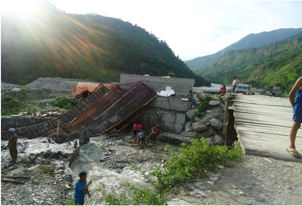
Fig. 5 b: The labours are stock piling the formworks and reinforcements which were washed away by the flood. The concrete abutment at right side which was recently completed can be seen on photo. The condition of both abutments is good.
