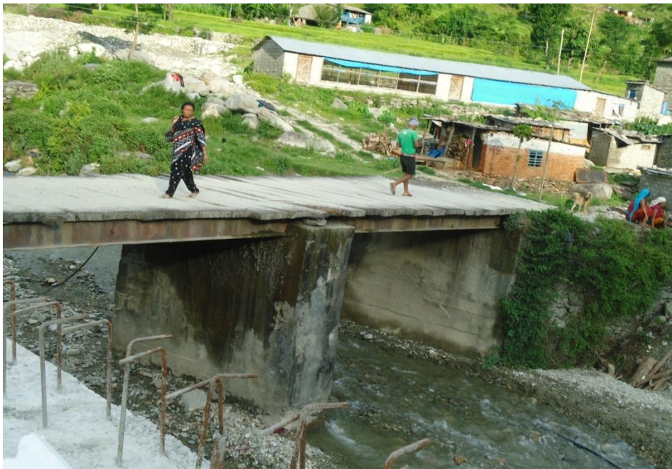
Fig.5c: Existing temporary wooden (motorable) bridge. This bridge is located at about 15 m upstream from the damaged bridge. At present all the vehicles and pedestrians use this bridge for crossing.
