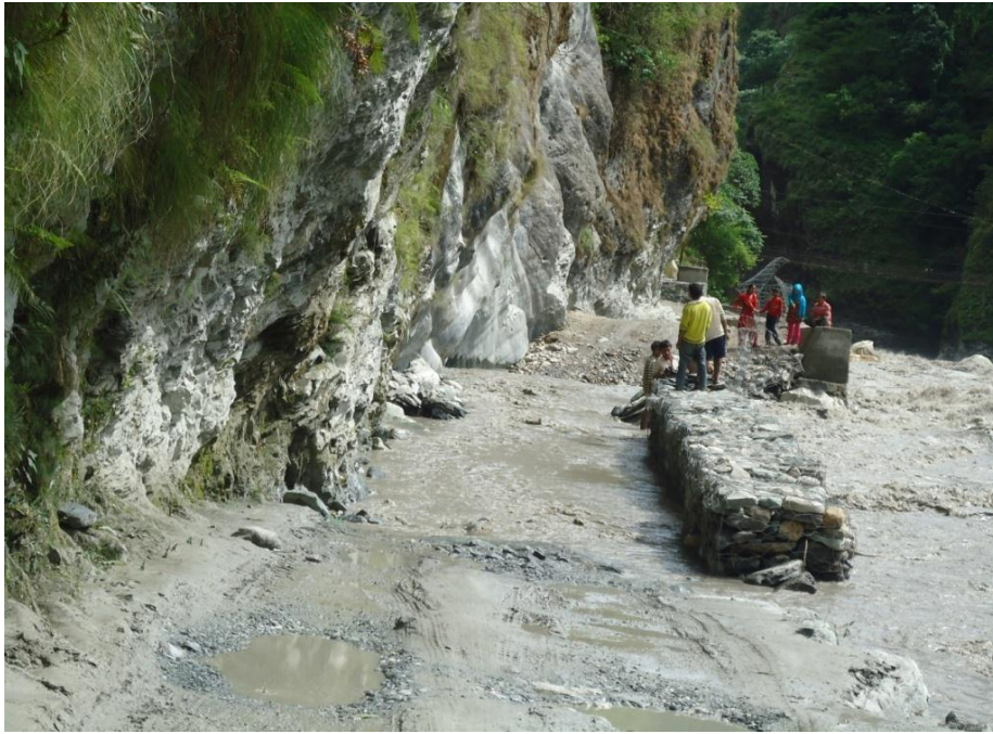
Fig.4a Damaged section of the road at km 17. The damage occurred due to extensive bank erosion by Kaligandaki River. At present, DoR is constructing gabion wall to protect the road from river damage.
