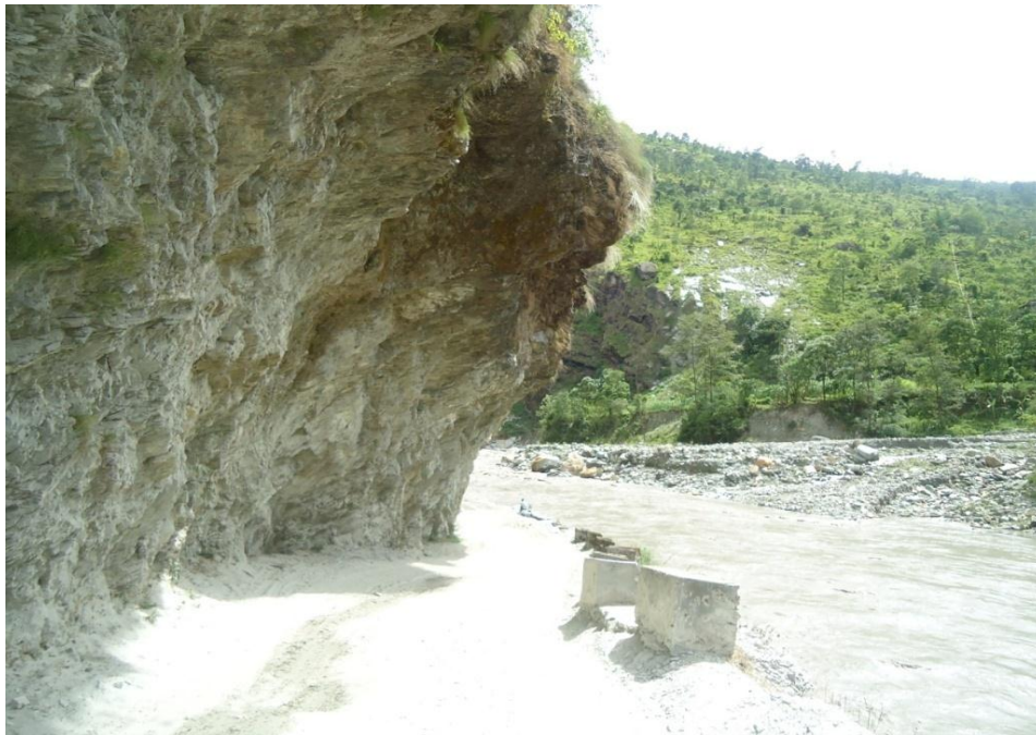
Fig.4b At right side of the photo, the heap of gravels and boulders is the debris deposited by Sunari Khola in July 2013. The debris pushed the River towards left bank and severely damaged the road.
