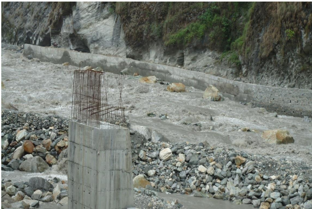
Fig. 4d: Photo of newly constructed wall to protect the road which is located at left bank. The photo is taken from right bank. DoR has already constructed about 100 long stone masonry/concrete protection walls and reconstructed damaged road section. DoR is constructing a motorable bridge near the damaged road. Right abutment of the bridge is also seen on photo.
