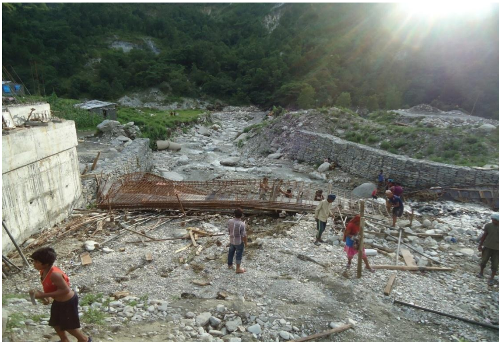
Fig. 5a: View of the bridge after the flood washed away formworks, struts, and reinforcements. Upstream view of the khola is also seen on photo. The photo was taken after 3 days of the event. As seen on photo, the khola has already dried up.
