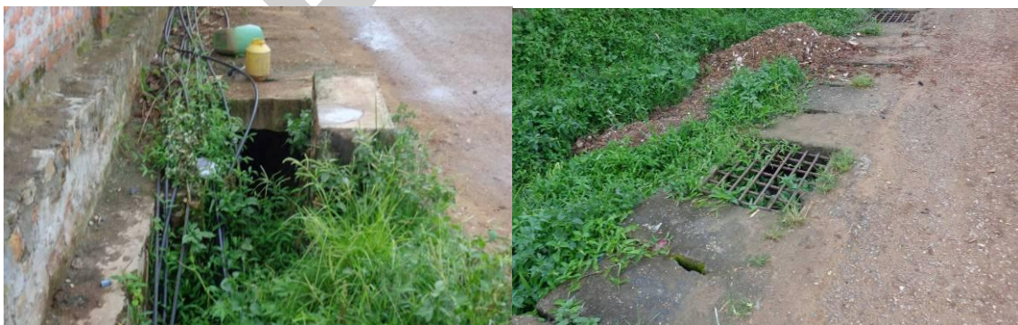
Figure 3.10: The existing condition of the old drains.
