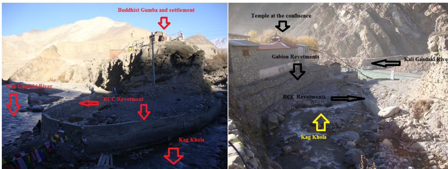
Fig. 3.1.2 Bank Protection works at the confluence of the Kag Khola and the Kali Gandaki rivers at Kagbeni.
