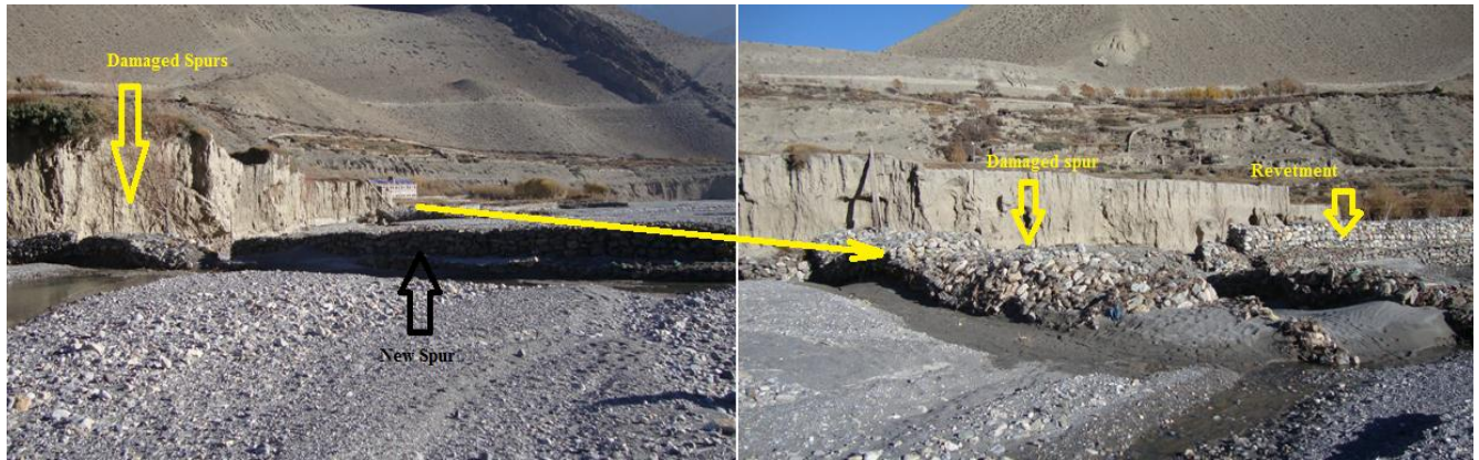
Fig. 3.1.3 Bank protection works along left bank of the Kaligandaki river d/s of the junction
