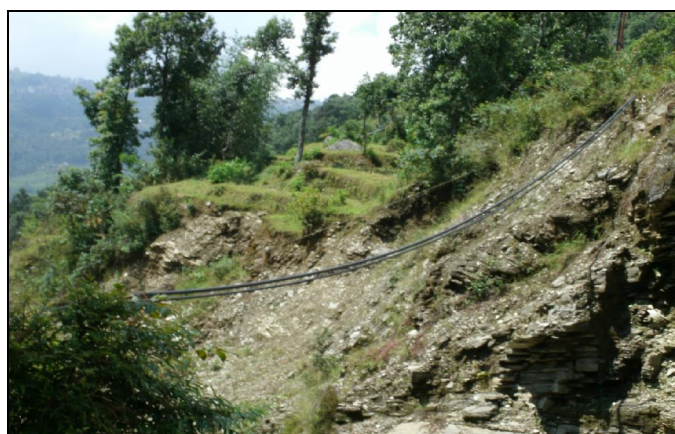
Figure 3-1: Hanging transmission pipeline along the historic landslide area
