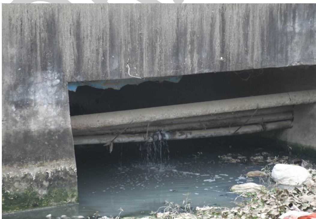
Figure 3-2 Pipe leakage and cross-contamination area
