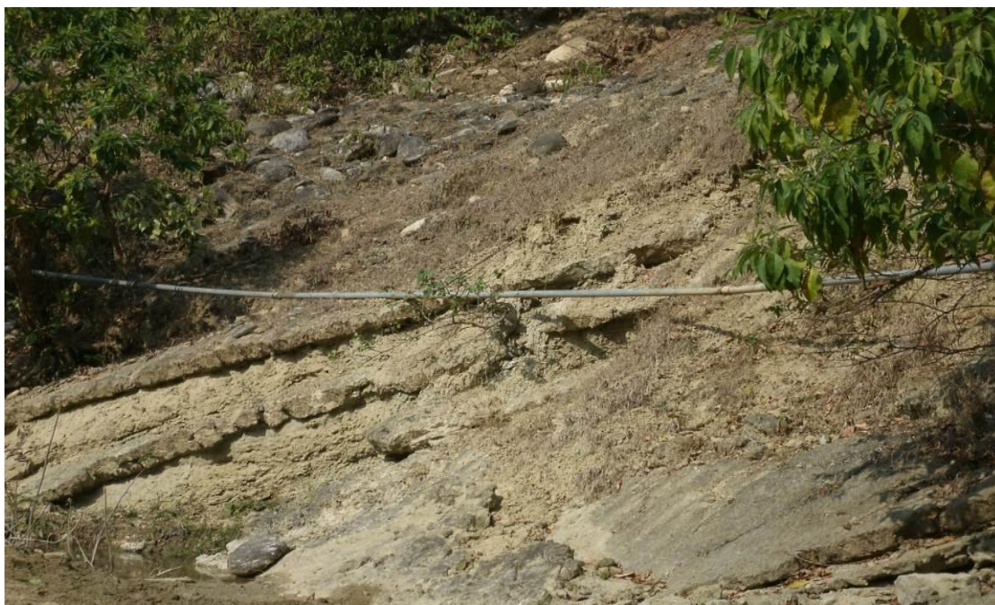
Figure 3-7: Khokari transmission pipeline exposed along stream bank
