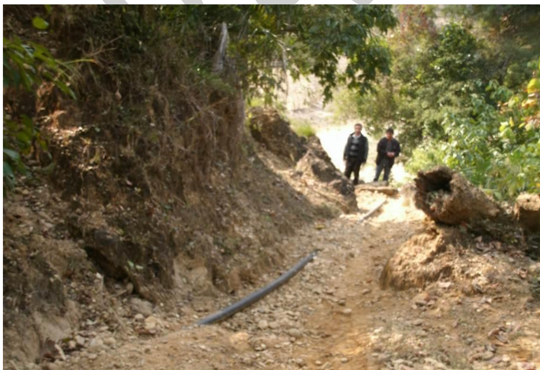
Figure 3-8: Khokari transmission pipeline exposed to open environment
