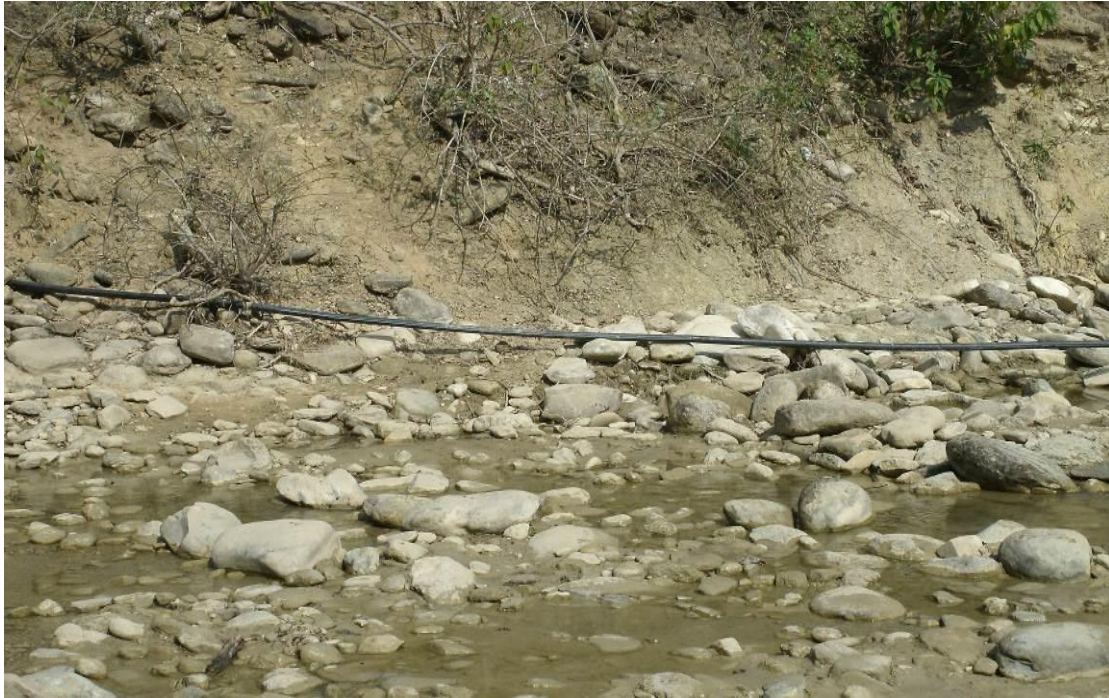
Figure 3-9: Khokari transmission pipeline exposed to open environment
