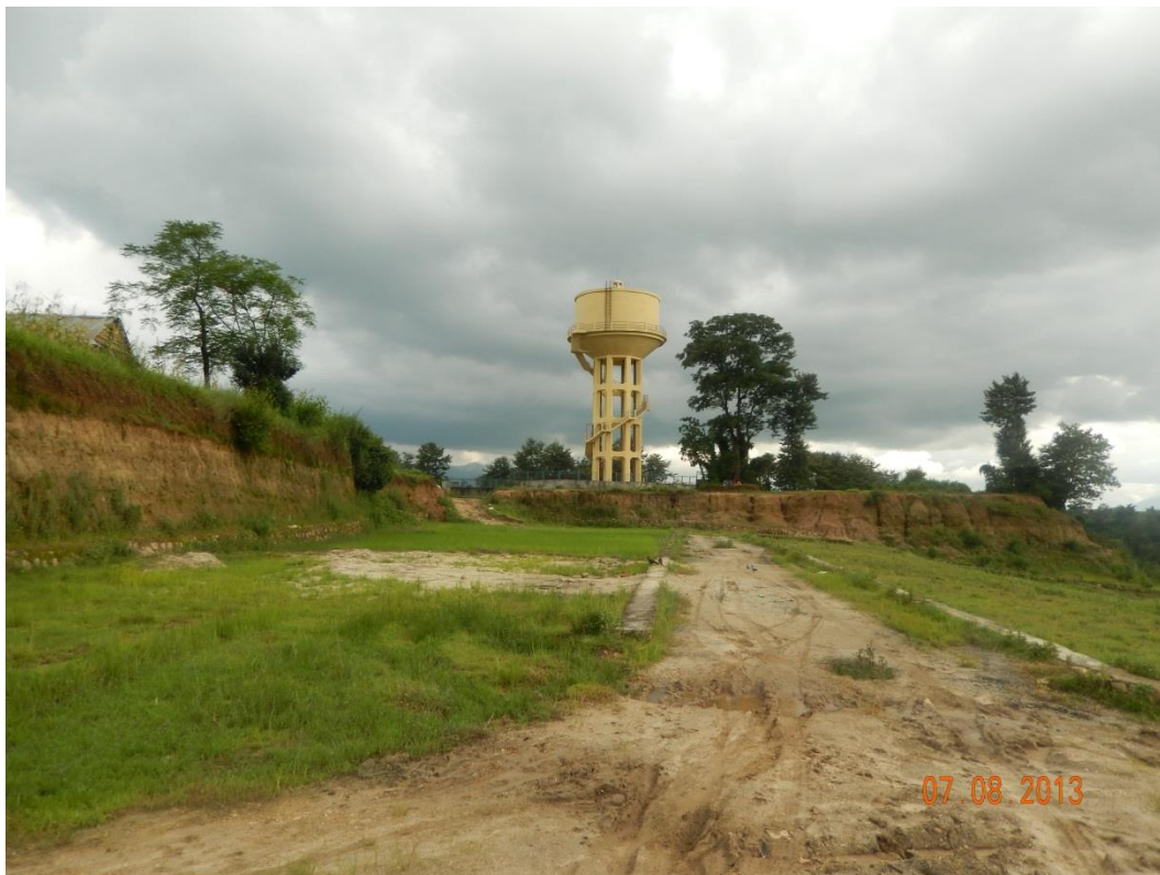
Figure 3-3: Overhead tank constructed on historic landslide area
