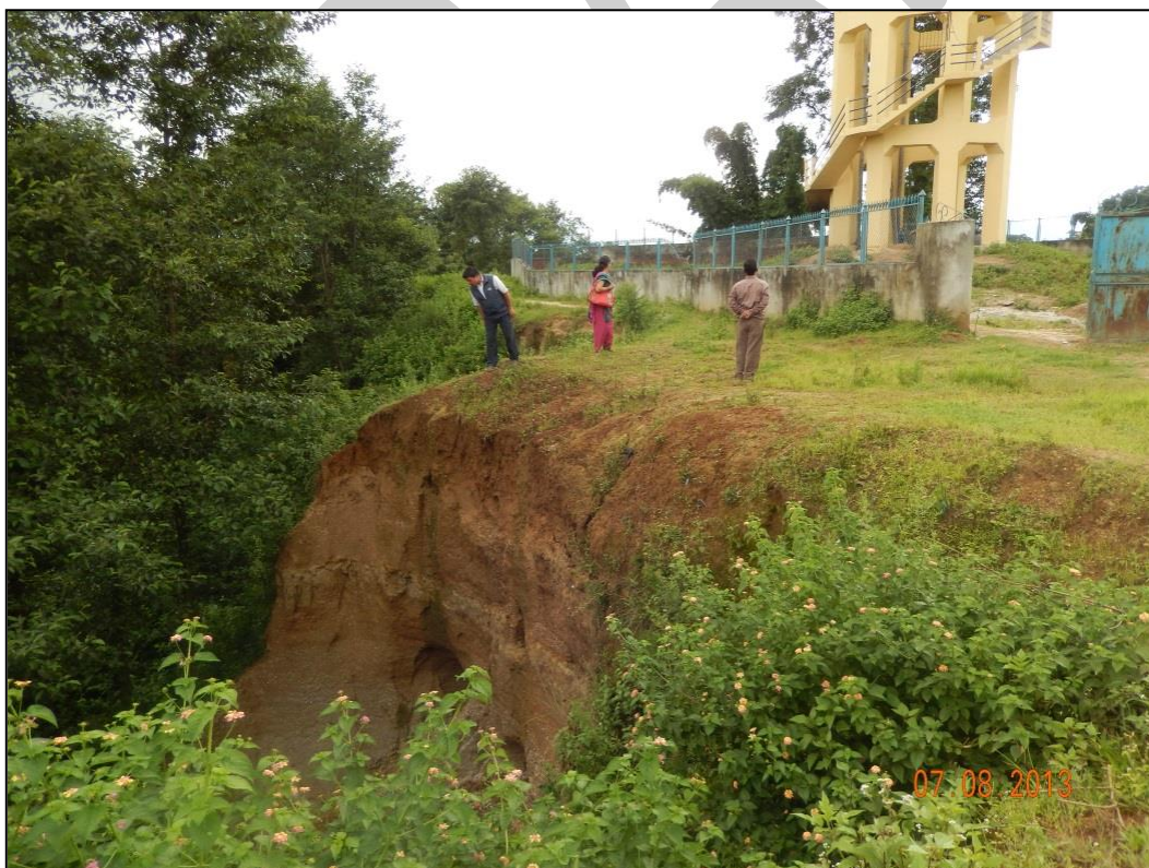
Figure 3-3: Overhead tank constructed on historic landslide area
